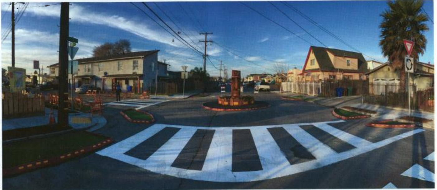
The quick build traffic circle includes a centerpiece totem pole as a gateway to the Pogo Park area in Richmond, CA, USA.
