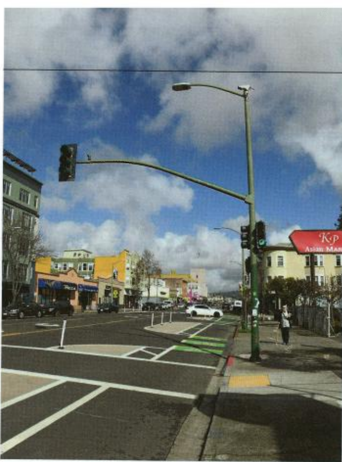
Telegraph Avenue's painted islands were an interim design project as part of the project's short-game plan.
