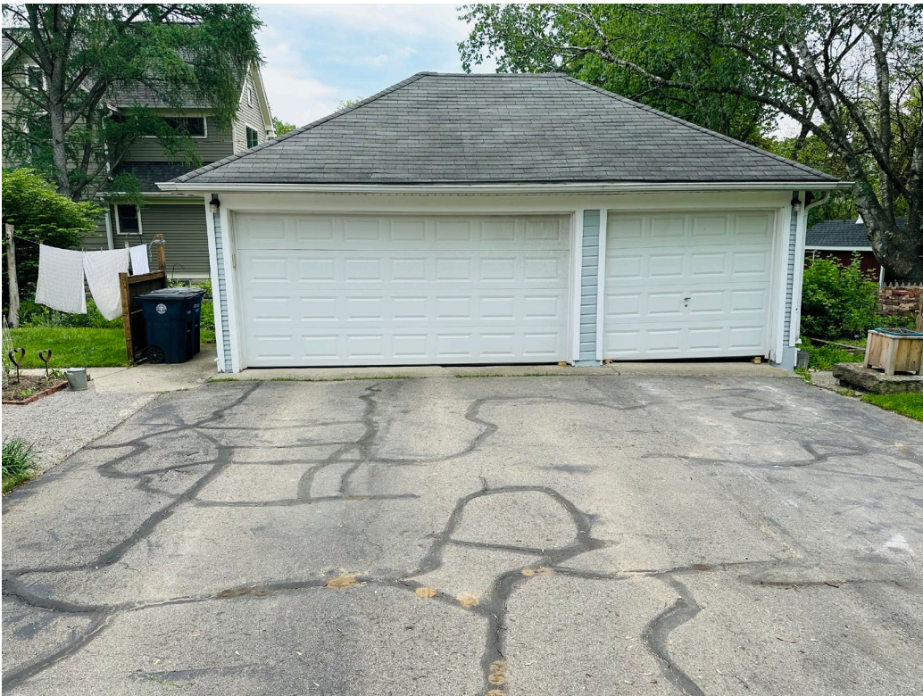
719 West Jefferson St, garage and paved driveway, 2024 (courtesy of applicant)
