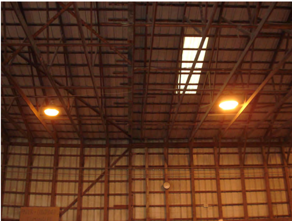
6. Trusses slope downward from the north to the south wall.
