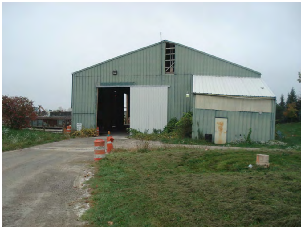
4. East end of building.
