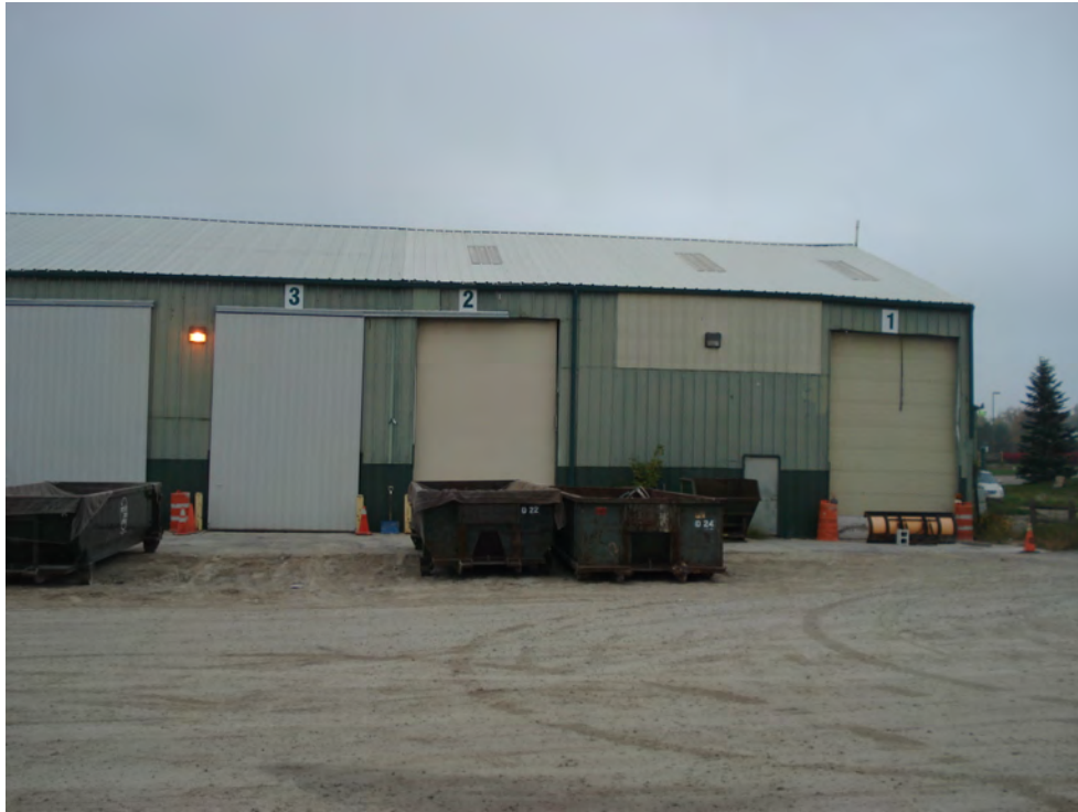
3. Front of building, east end.
