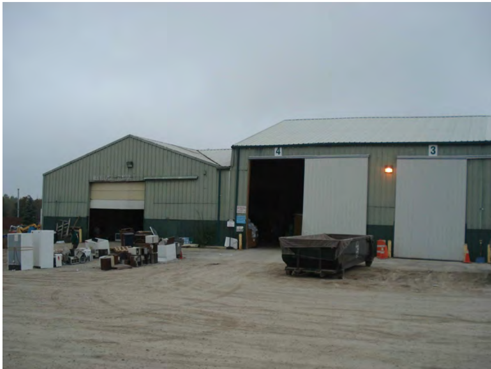
2. Front of building, west end.
