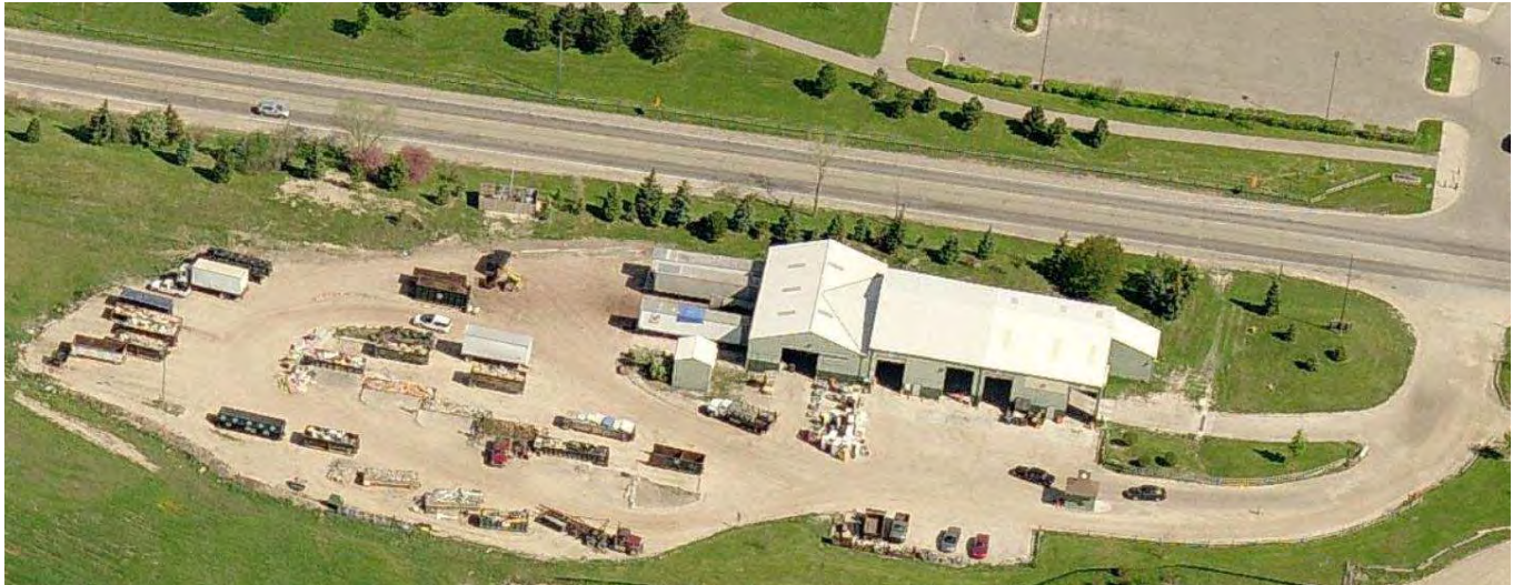
1. Aerial photo from Microsoft BING taken in about 2007. Building faces south.
