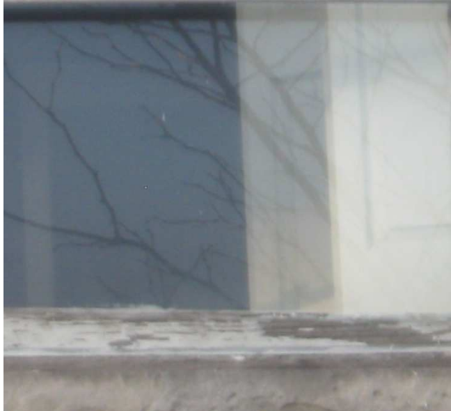
Closeup of Window 5
