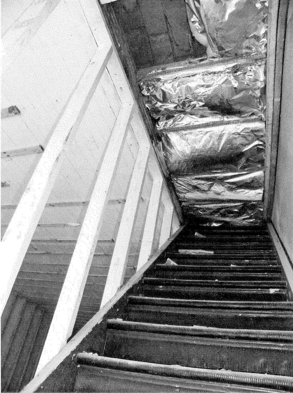
The original stairs to the former second and third floors still exist within the remaining single story Running Fit Building.
