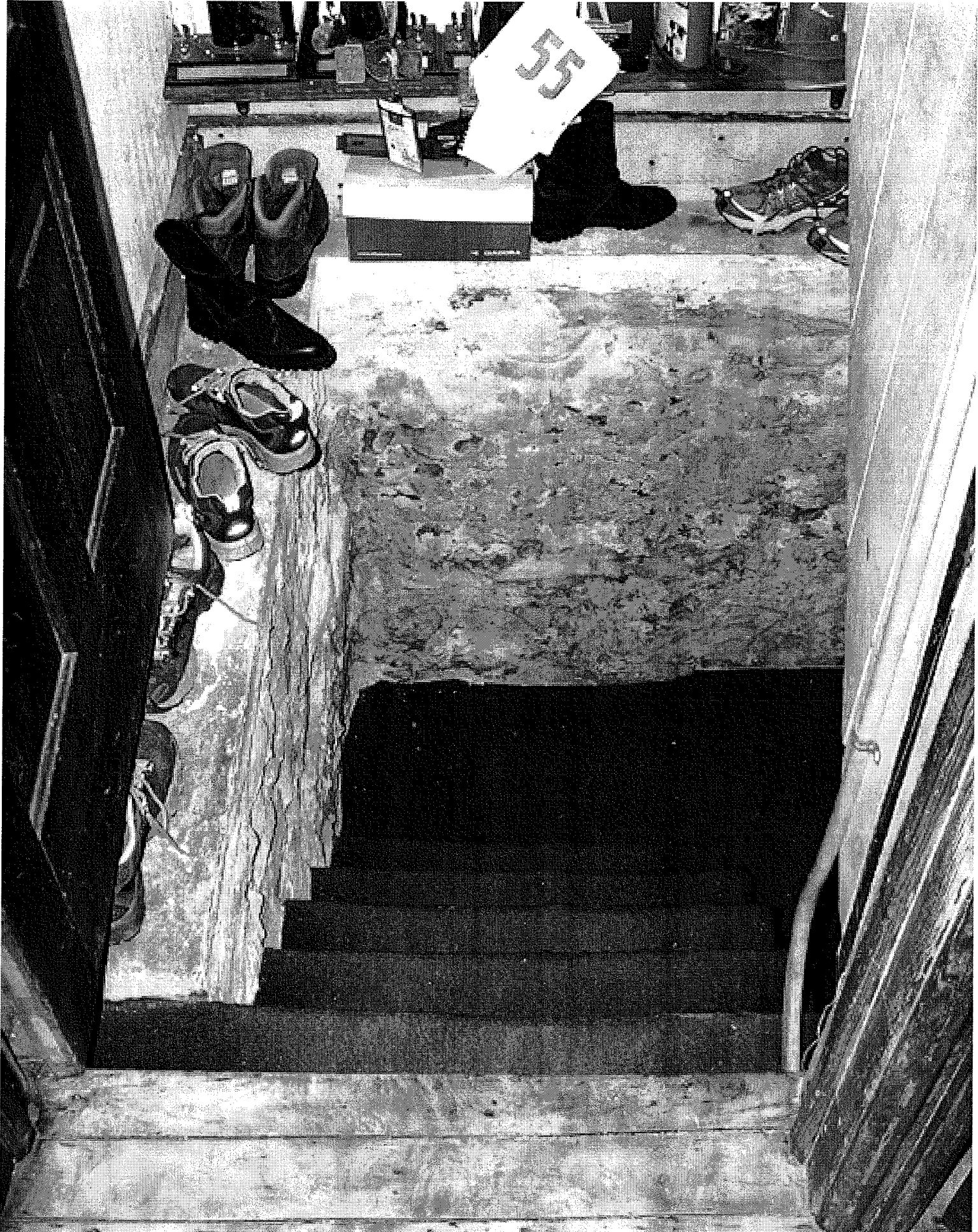
Basement Stair from Dining Room
