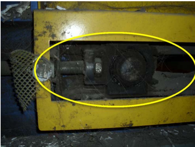
Bearing is worn, guarding is omitted, replacement required.
