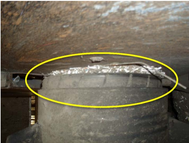
Picture shows belt tracking being off.
