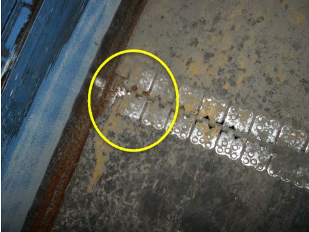
Belt and lacing is torn and needs to be replaced.
