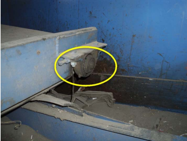
Bearing is worn, replacement required.
