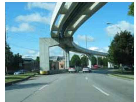
The concrete rails of the guideway are designed with a gap between them to combat winter snow accumulation
