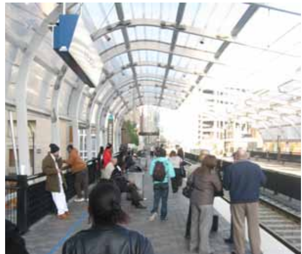
Stations feature passenger canopies for protection during poor weather conditions
