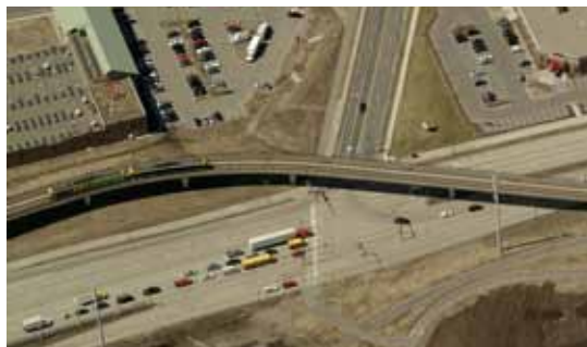
Elevated grade separations and a tunnel into the airport provide travel time advantages
