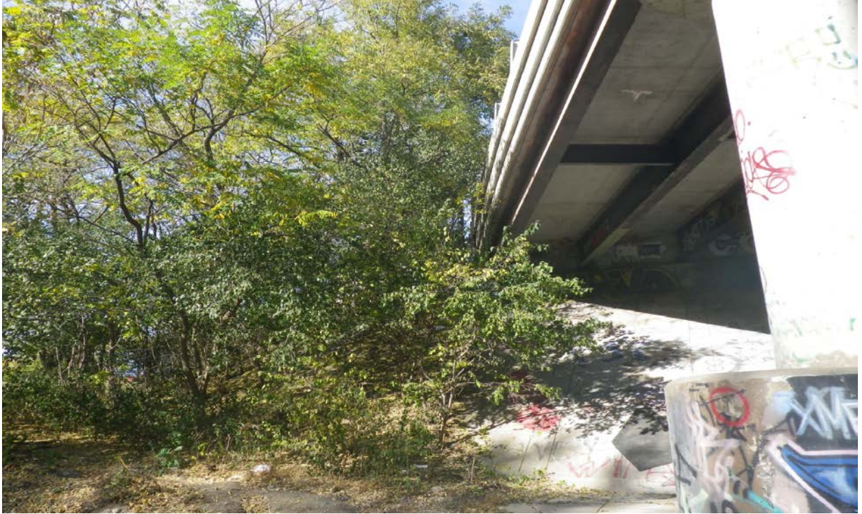
Figure 15 Typical heavy vegetation surrounding bridge
