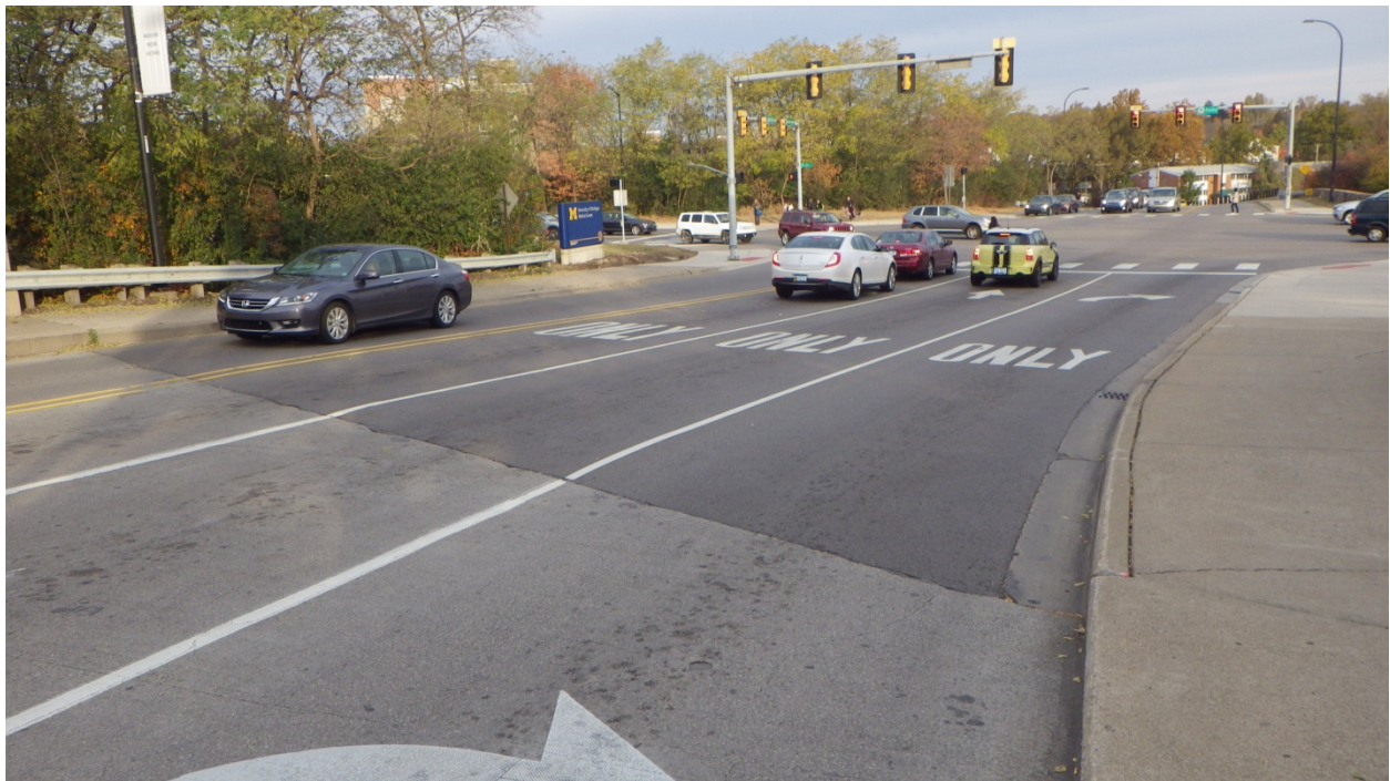
Figure 8 North Approach (looking north)
