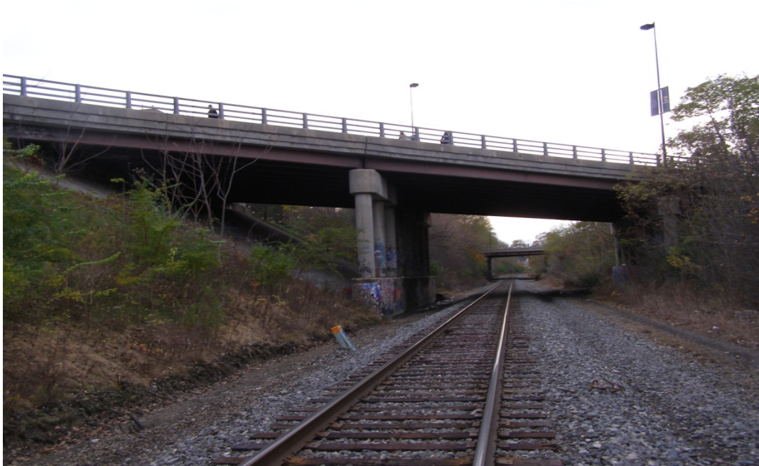
Figure 1 East Elevation Looking West
