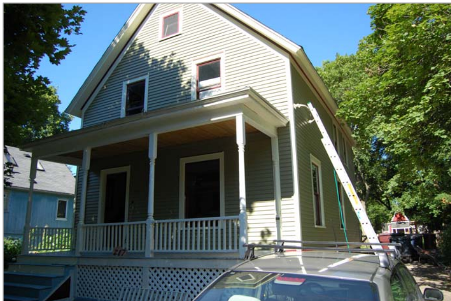
217 S Seventh Street (August 2010, courtesy of the applicant)
