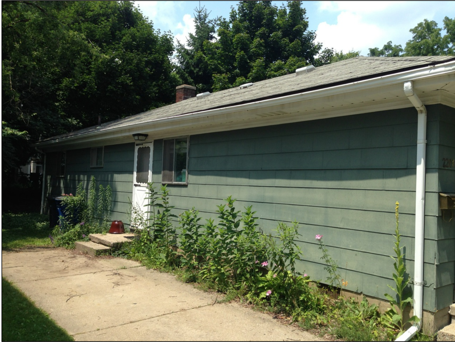
Current south side – 220 ½ Buena Vista Ave.
