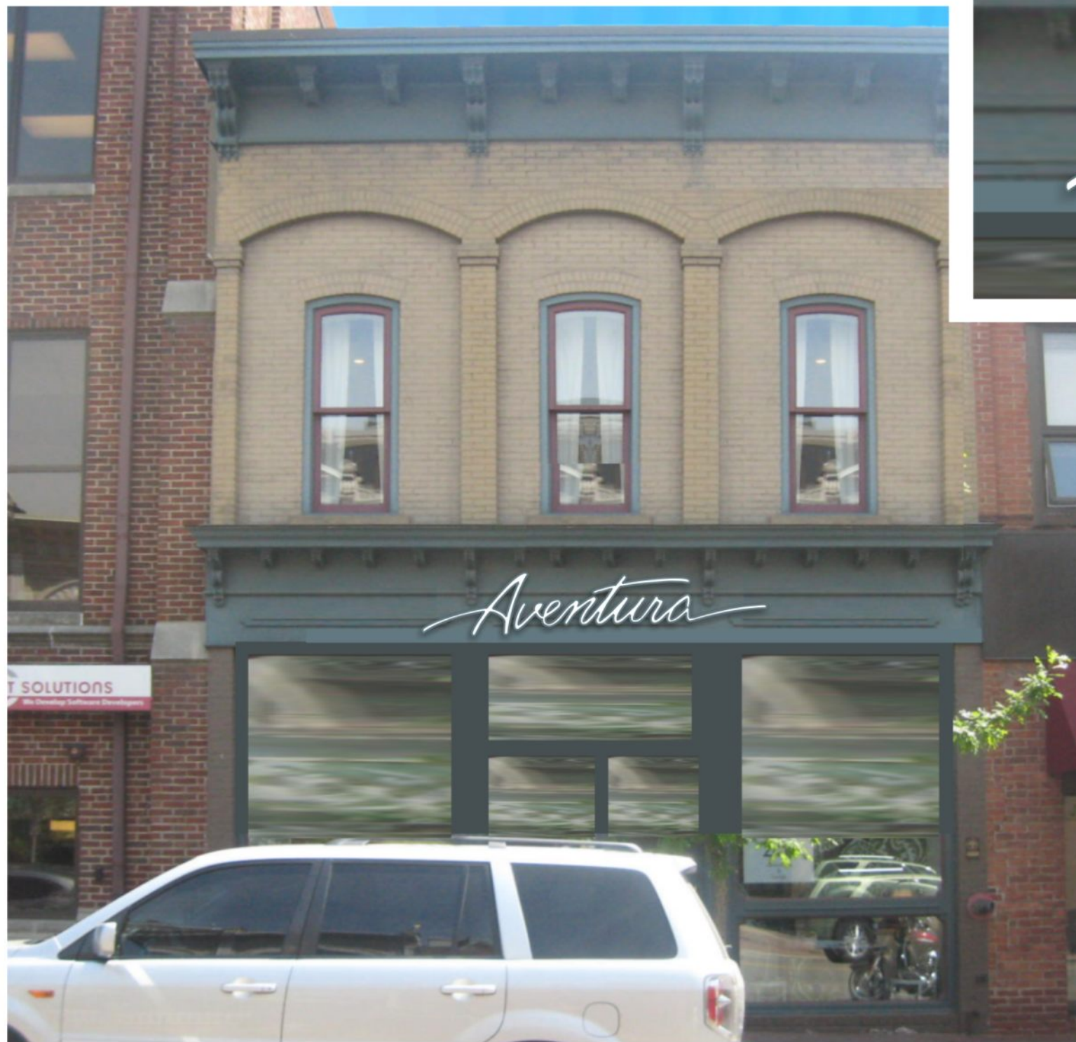
SURFACE MOUNTED NEON SIGN WITH REMOTE TRANSFORMER
