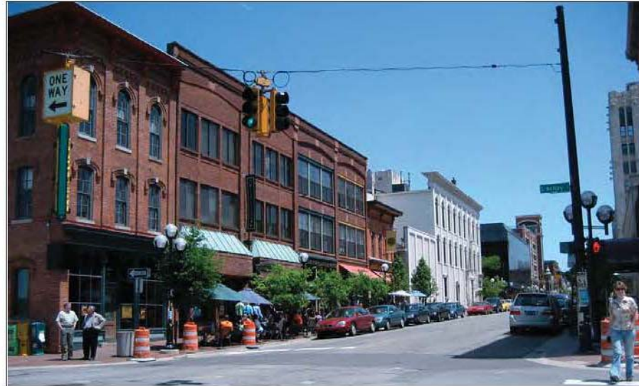
The established two- to three-story streetwall height within most parts of the Main Street character area and historic district should be maintained.
