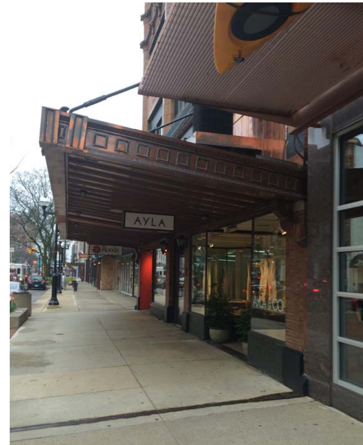
Moosejaw canopy south of Whitker Building
