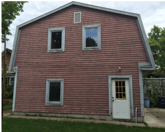
TOP PHOTO OF ORIGINAL 2 STORY HOUSE WITH ADDITION AT REAR WITH DECKS. BOTTOM PHOTO OF ORIGINAL 2 STORY GARAGE SOUTH SIDE.
