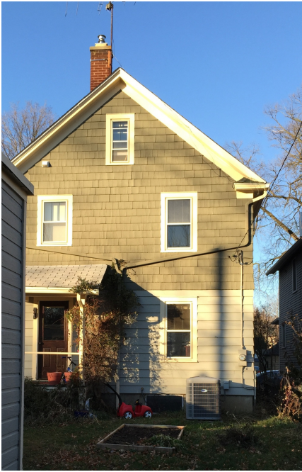
CHIMNEY TO BE REMOVED & ATTIC WINDOW TO BE REPLACE (REAR)
