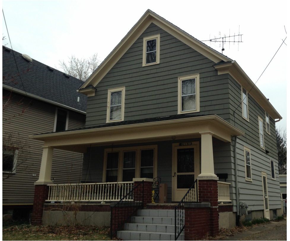
VIEW OF NORTHWEST CORNER FROM SIDEWALK (CHIMNEY AT BACK OF HOUSE NOT VISIBLE, SIDE BASEMENT WINDOWS TO BE REPLACED, ATTIC WINDOW TO BE REPLACED)
