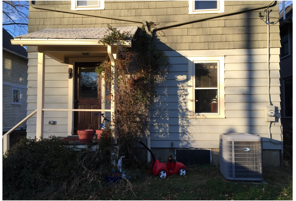
REAR BASEMENT WINDOW TO BE REPLACED
