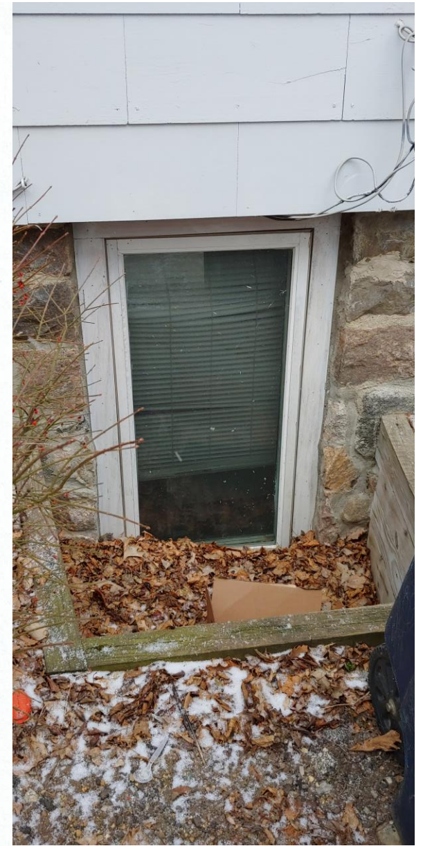
Example of Anderson casement window with wood trim and wood window well
