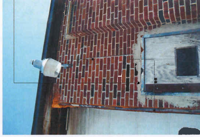
W1.3 The existing brick and mortar joints appear to be in poor condition. In many areas the mortar has completely deteriorated and the brick has spalled and cracked away. The brick facade is penetrated by pipes and conduit with no joint sealant around the perimeter of the opening.
