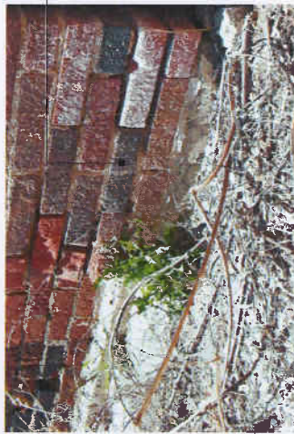
E1.2 The existing brick and mortar joints appear to be in poor condition in concentrated areas along the base of the building. In many areas the mortar has completely deteriorated and the brick has spalled, flaked and cracked away. In some areas the bricks have come completely loose and have exposed the inner wall cavity to both air and water infiltration.
