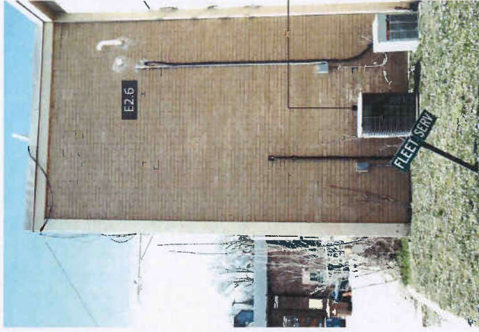
E2.2 The existing brick veneer and mortar joints appear to be in good-to-fair condition with minor signs of deterioration at the base of the steel column above the concrete foundation wall. The joint sealant between the brick and steel column has cracked and opened in many areas. The inner wall cavity has been exposed to both air and water infiltration.
