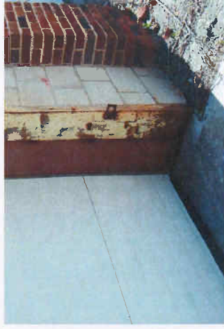
W1.2 A section of the existing steel window sash and glazing has been removed to accommodate the installation of a louvered vent. A sheet of untreated, moderately deteriorated plywood creates a perimeter seal at the glazing opening. Sealant between the steel sash and plywood sheathing has deteriorated.
