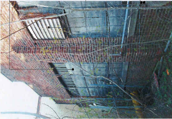
N1.1 Spray-on insulation has been applied to the existing steel sash windows, jambs, head and sill; bonding to the steel and glazing. The northern exposure, out-building and vegetation have protected the original fluid applied weather-resistant membrane, which remains relatively intact. Small sections of the spray on insulation are cut open and exposed.
