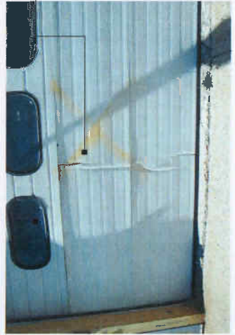
E2.3 Insulated face of the overhead door has been damaged in multiple locations. Weather stripping has broken away in many areas and the perimeter of the door has been breached by air and water infiltration. Adjacent key operator switch has been disconnected and signs of adjacent corrosion and deterioration were observed.
