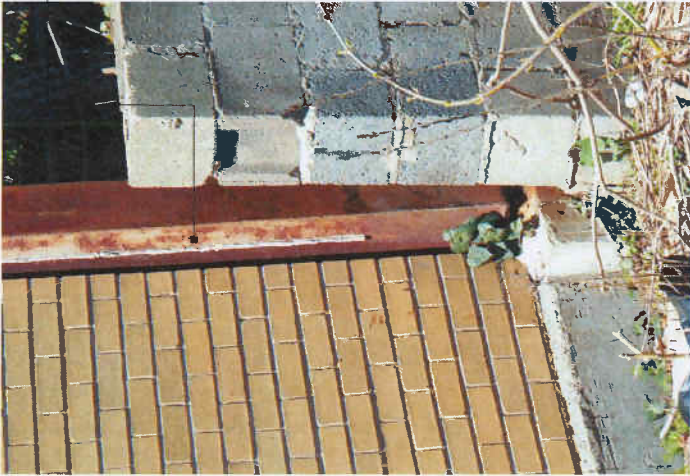
E2.1 Separation between the brick facade and steel column has occurred at NE corner of the building (see structural assessment for further evaluation). The resulting aperture between the brick and steel structure has caused separation of the joint sealant and exposed the internal cavity wall system to water, insect and air infiltration.
