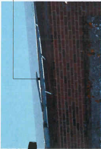
E1.1 The gutter has disconnected from hangers at many locations along the existing fascia. Several hangers have broken and fallen away from the building. The gutter is sagging and deteriorated in locations where water cannot drain.
