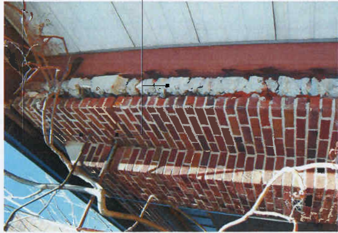
W1.3 The existing brick and mortar joints appear to be in poor condition. In many areas the mortar has completely deteriorated and the brick has spalled and cracked away. The brick facade is penetrated by pipes and conduit with no joint sealant around the perimeter of the opening.
