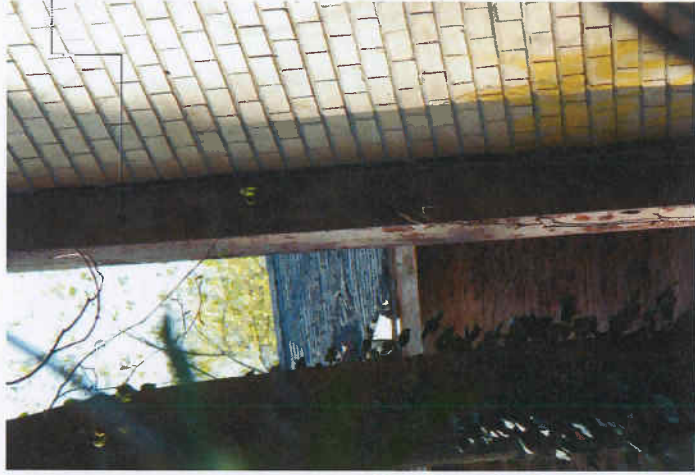
N2.1 Glazing is mostly covered with foam insulation panels that are rotted and blackened in color.
