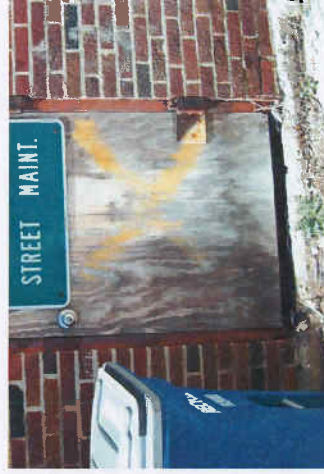
E1.2 The existing brick and mortar joints appear to be in poor condition in concentrated areas along the base of the building. In many areas the mortar has completely deteriorated and the brick has spalled, flaked and cracked away. In some areas the bricks have come completely loose and have exposed the inner wall cavity to both air and water infiltration.
