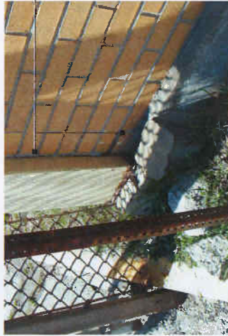
E2.2 The existing brick veneer and mortar joints appear to be in good-to-fair condition with minor signs of deterioration at the base of the steel column above the concrete foundation wall. The joint sealant between the brick and steel column has cracked and opened in many areas. The inner wall cavity has been exposed to both air and water infiltration.
