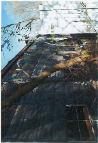
N2.1 Glazing is mostly covered with foam insulation panels that are rotted and blackened in color.
