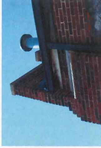
E1.1 The gutter has disconnected from hangers at many locations along the existing fascia. Several hangers have broken and fallen away from the building. The gutter is sagging and deteriorated in locations where water cannot drain.
