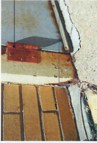
E2.1 Separation between the brick facade and steel column has occurred at NE corner of the building (see structural assessment for further evaluation). The resulting aperture between the brick and steel structure has caused separation of the joint sealant and exposed the internal cavity wall system to water, insect and air infiltration.
