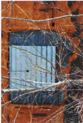
W1.2 A section of the existing steel window sash and glazing has been removed to accommodate the installation of a louvered vent. A sheet of untreated, moderately deteriorated plywood creates a perimeter seal at the glazing opening. Sealant between the steel sash and plywood sheathing has deteriorated.
