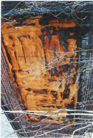
W1.1 Typical Window Bay; Spray-on insulation has been applied to the existing steel sash windows, jambs, head and sill; bonding to the steel and glazing. The original fluid applied weather-resistant membrane has deteriorated exposing the spray-on insulation to the elements. Original application of the fluid applied membrane has left staining on the concrete window sills and adjacent face brick.
