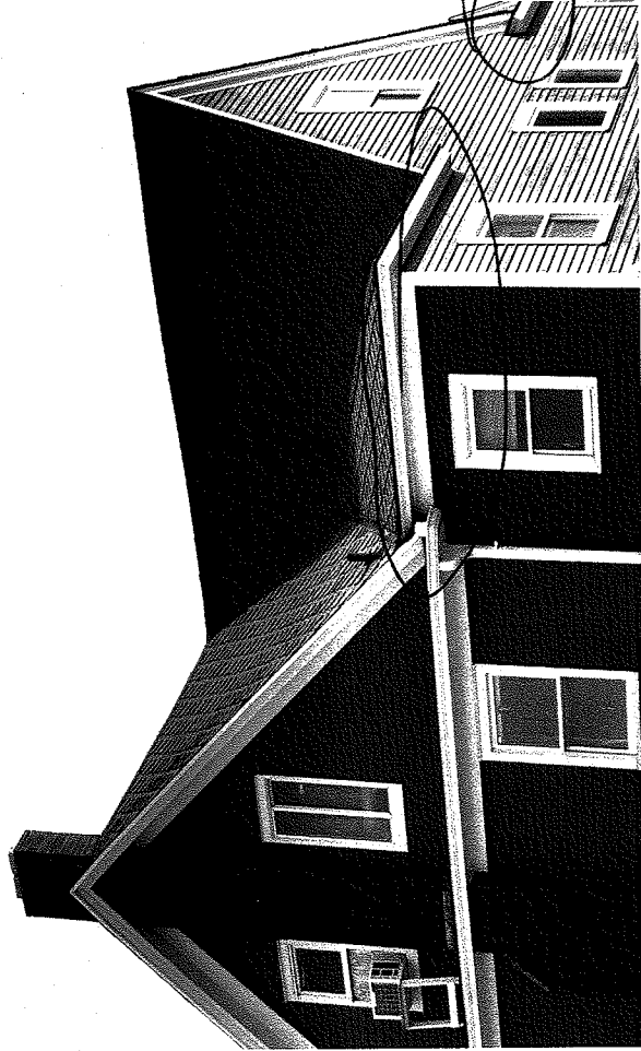
REAR 2ND STORY WEST FACING CONTINUOUS SOFFIT VENTING
