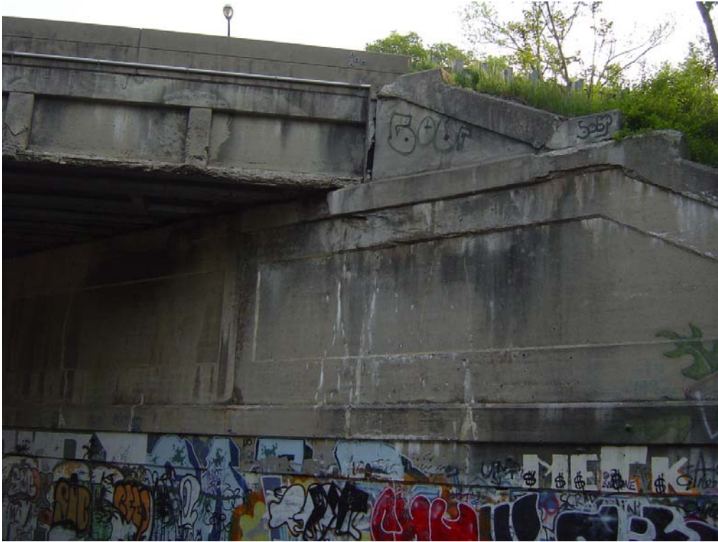
Bridge over railroad 300 feet west of the State Street Bridge
