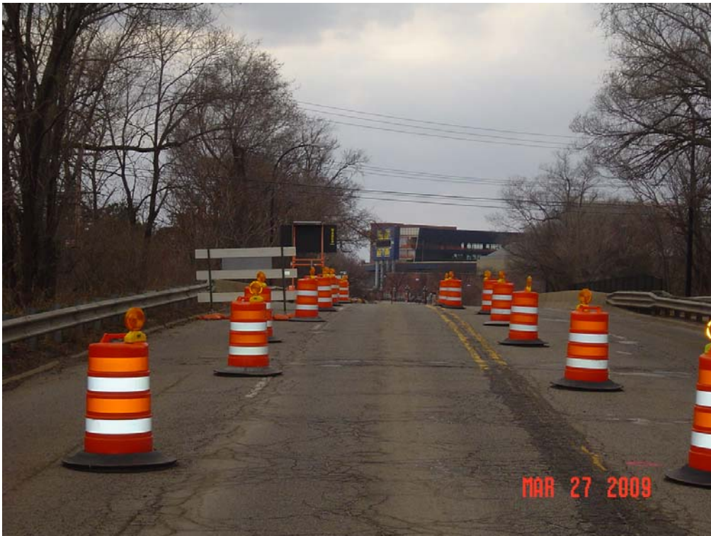
Traffic control on Stadium Bridge over State Street
