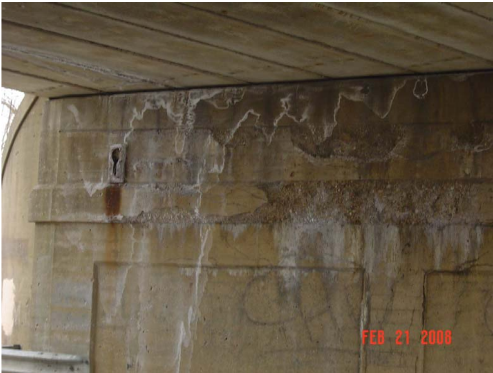
Condition of side walls of Stadium Bridge over State
