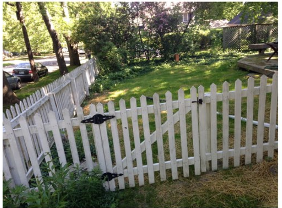
Another look at next door neighbor's fence (Fifth Street visible at left) with 2.75-inch pickets and gate to yard.
