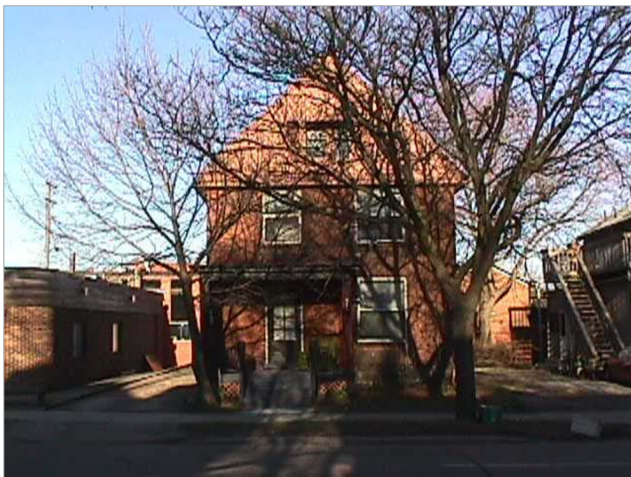
217 North Fifth Avenue (1999 Assessor's photo)
