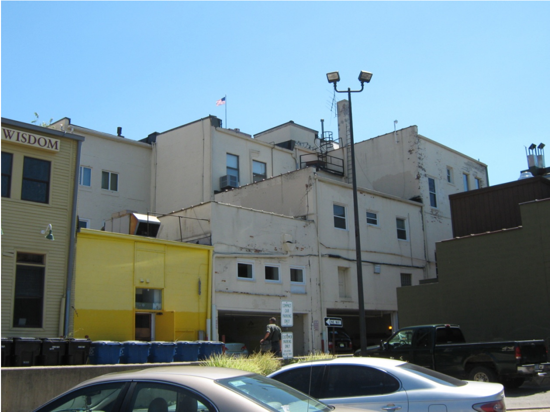
Rear view of 118-124 South Main (the three beige sections)
