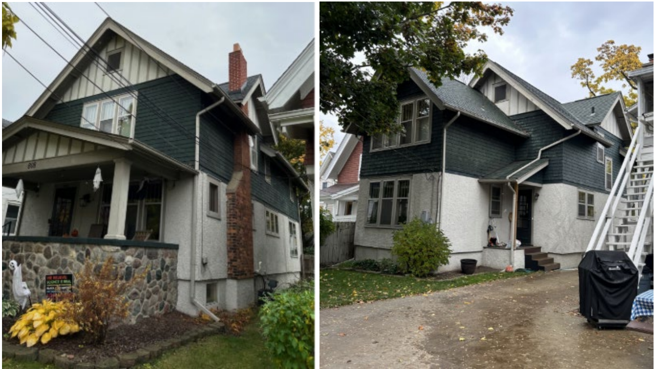
808 Lawrence Street, left: front, right: rear, 2024 (courtesy of applicant)
