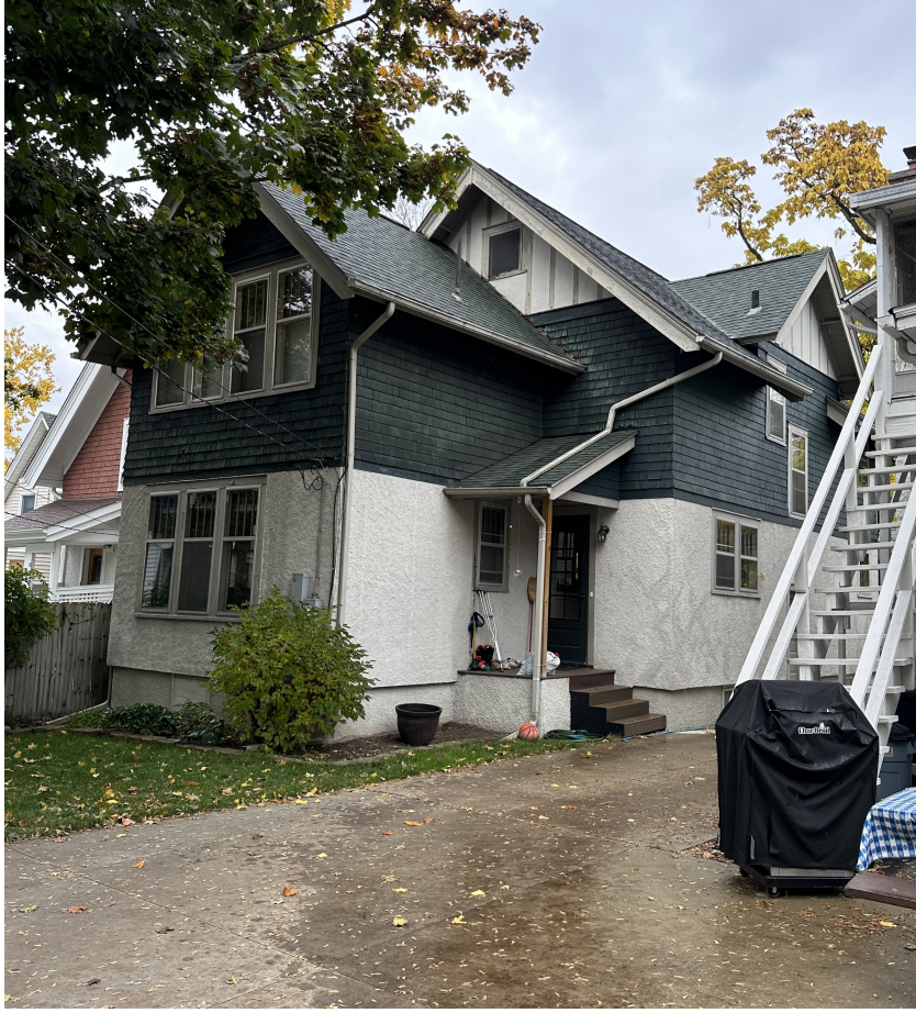
PHOTO OF EXISTING CONDITIONS REAR PORCH TO BE REMOVED
