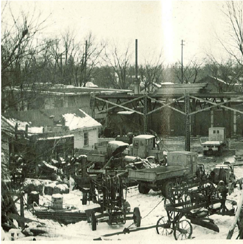
Photo showing construction of the steel framed high bay space
