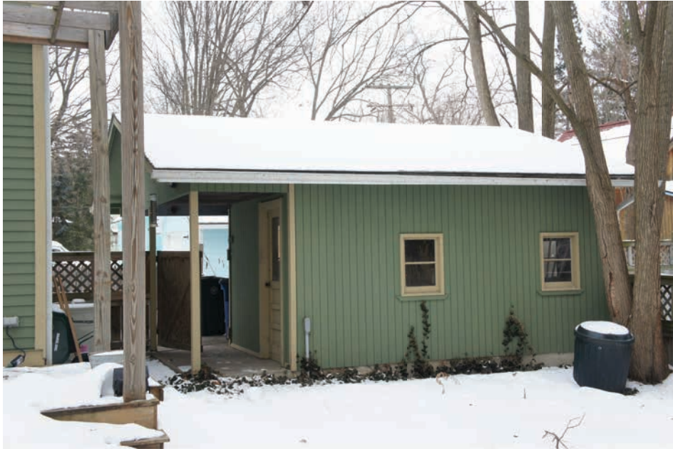
PHOTO: Existing 1969 1 Story Garage - south side.
