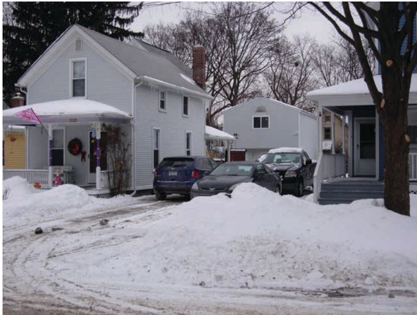
PHOTO: 533 Second St 2 Story House - Street view 2 Story wood Garage.
