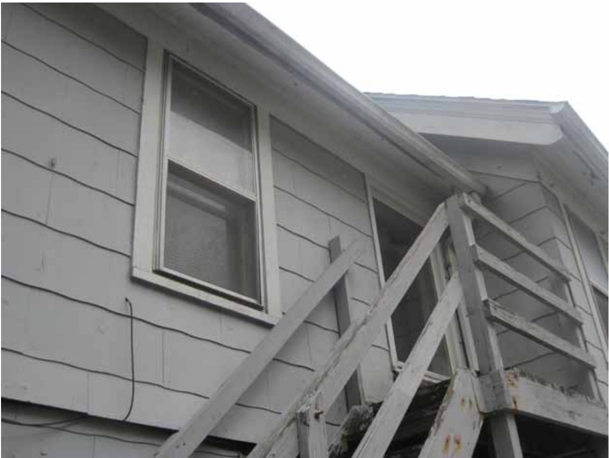
picture 6: Existing Wood Egress Stairs
