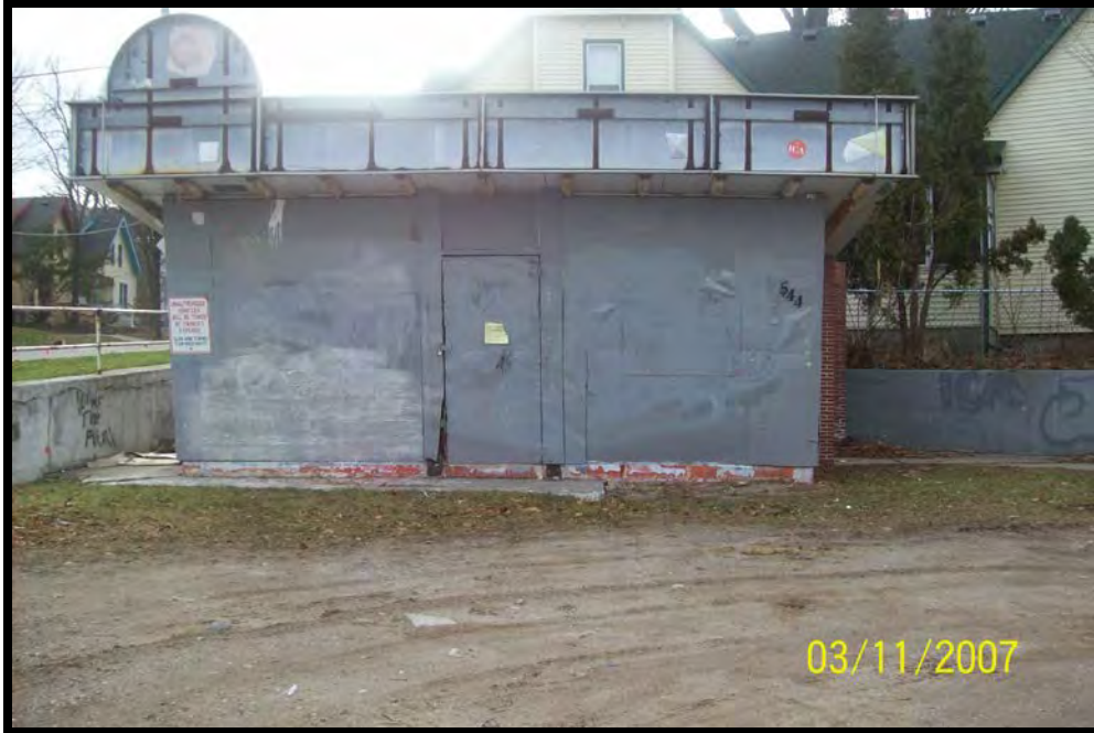
PHOTOGRAPH NO. 1: SUBJECT PROPERTY NORTHERN PORTION OF THE SUBJECT BUILDING
