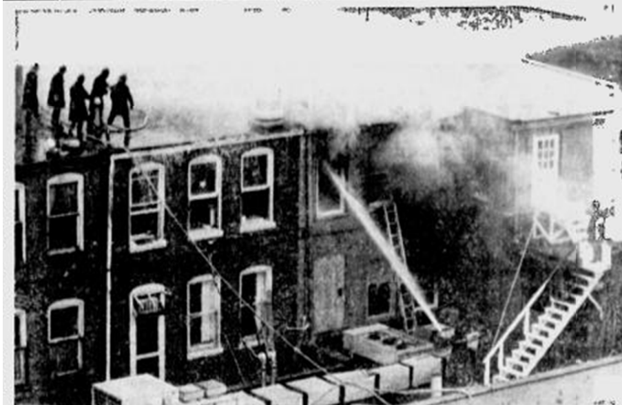
FIREFIGHTERS ATTEMPT to douse the blaze atop the Old German Restaurant. The fire gutted the downtown landmark and damaged several neighboring businesses as well. No one was seriously injured.
