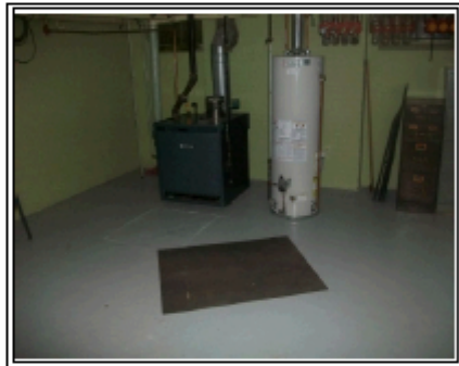
utility room in basement
