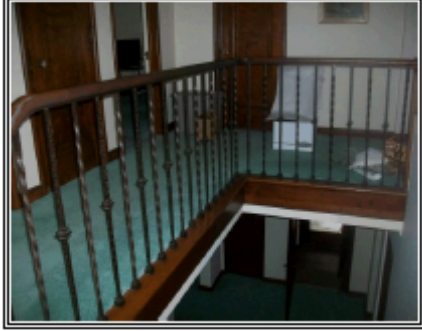
hall way second floor
