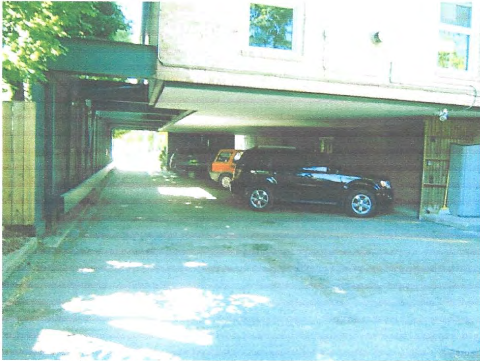
Looking at the covered parking from the rear of the site
