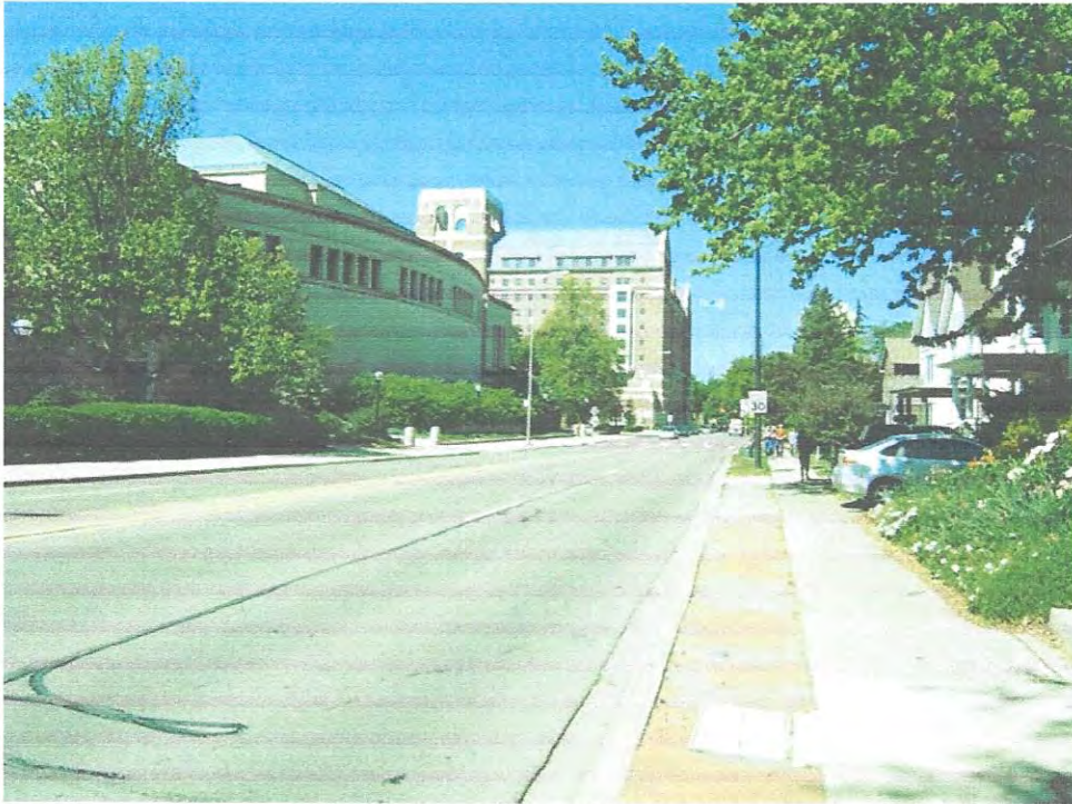
Looking west at Huron from the subject with Rackham Auditorium in view
