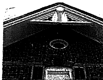
Fig. 12. West gable with stringcourse detail.
