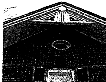
Fig. 12. West gable with stringcourse detail.
