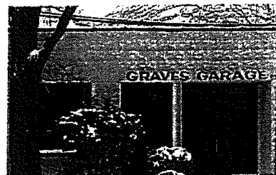
Fig. 2. East and middle bays.
