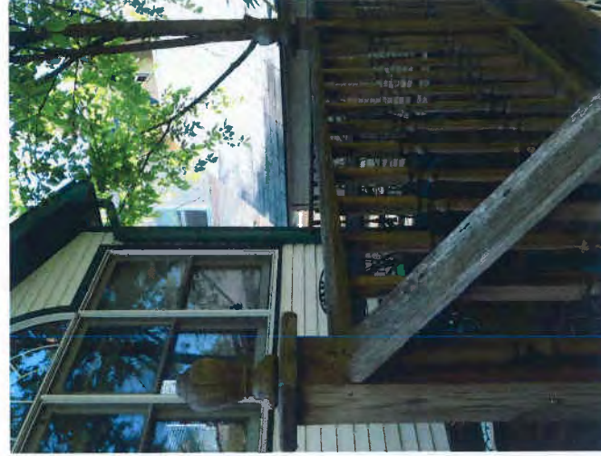
EXISTING DECK RAILING
