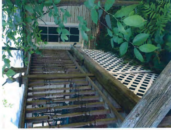
EXISTING DECK RAILING
