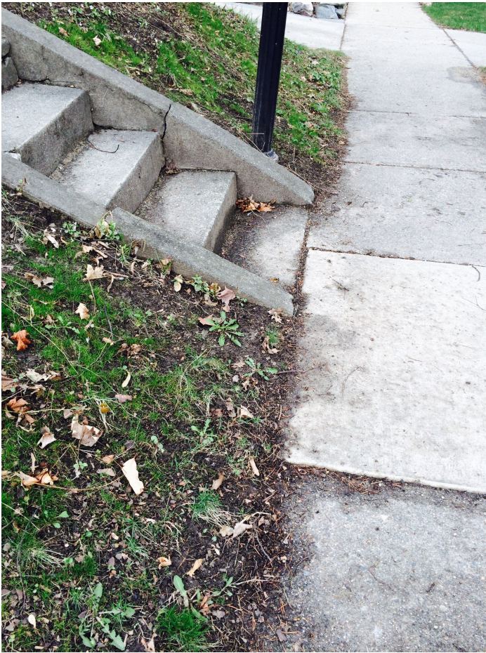
Existing Concrete Steps are cracking and deteriorating
