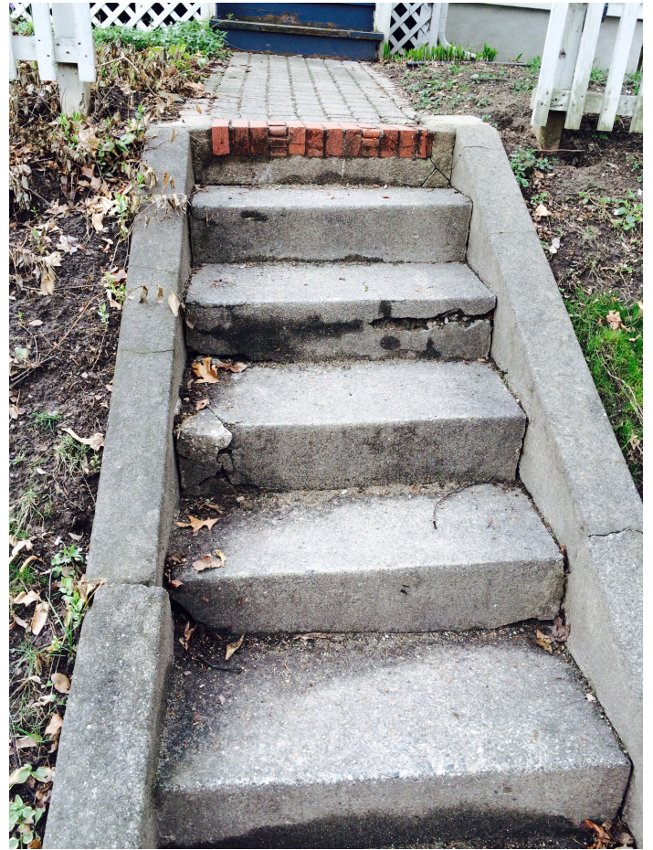
Existing Concrete Steps are cracking and deteriorating
