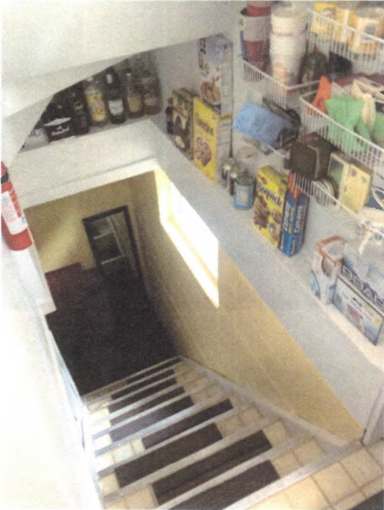
EXISTING BASEMENT STAIR
