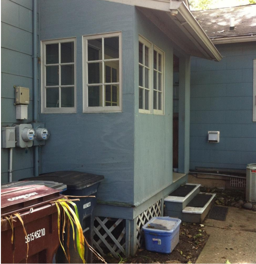
Photo 6. View from north.
