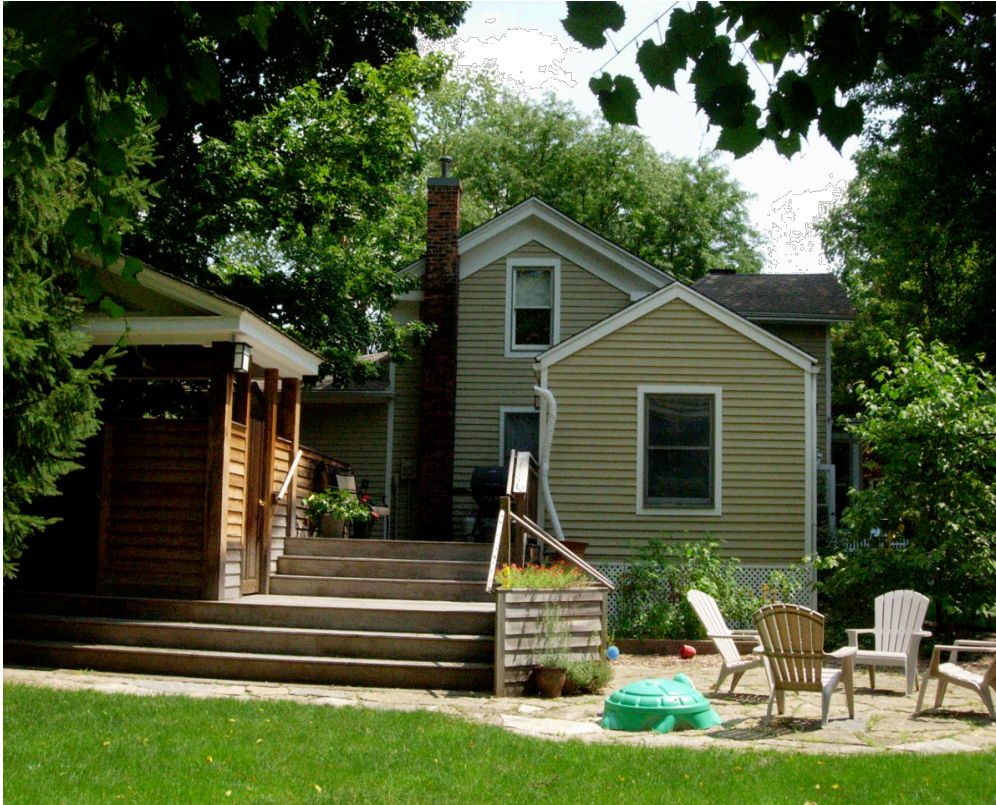
TOP PHOTO OF ORIGINAL 1 1/2 STORY HOUSE WITH 1980'S ADDITION AT RIGHT AND DECK WITH SAUNA AND HOT TUB STRUCTURE
