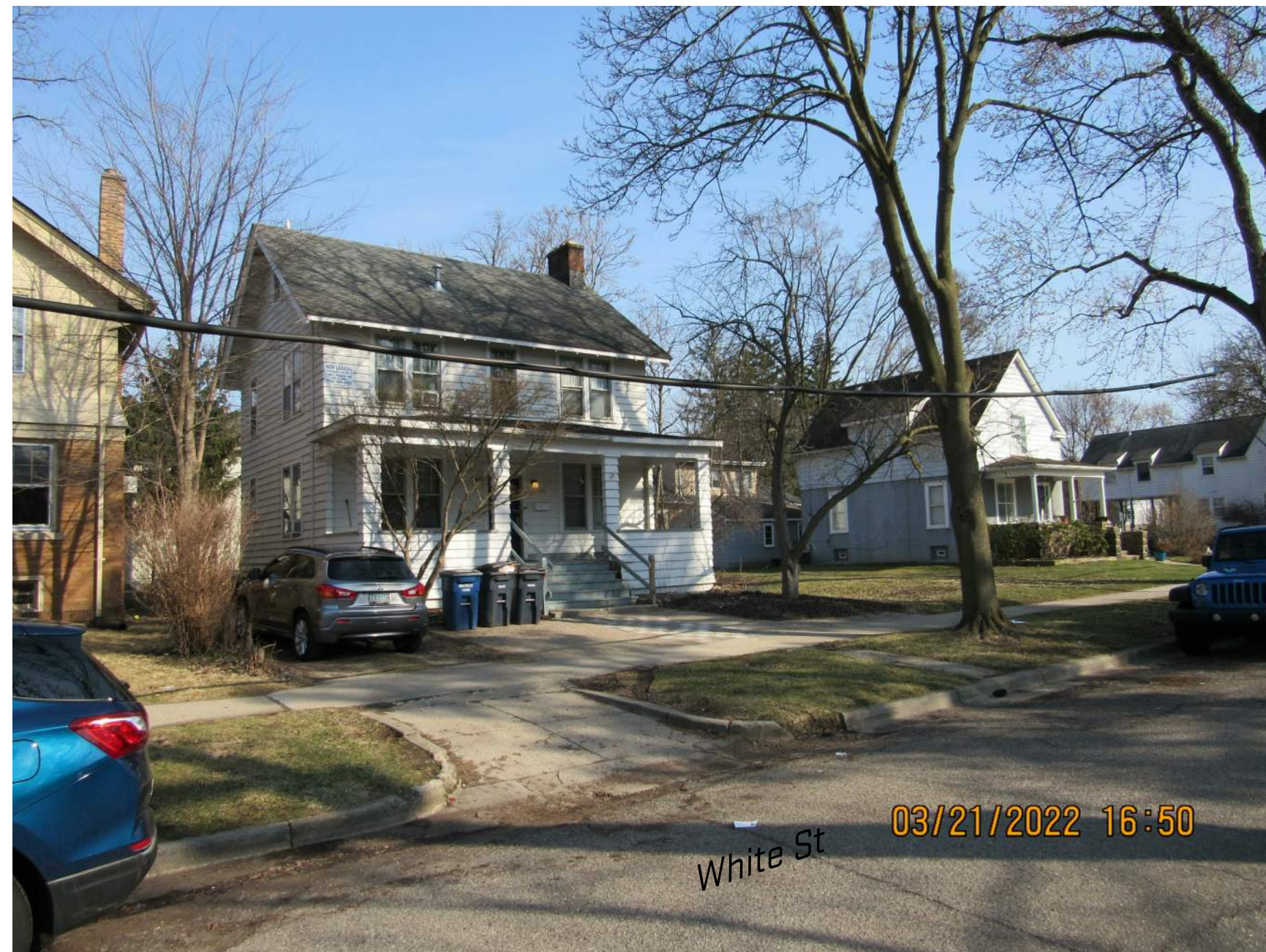
1203 White St / 1211 White St - NorthWest Facades
