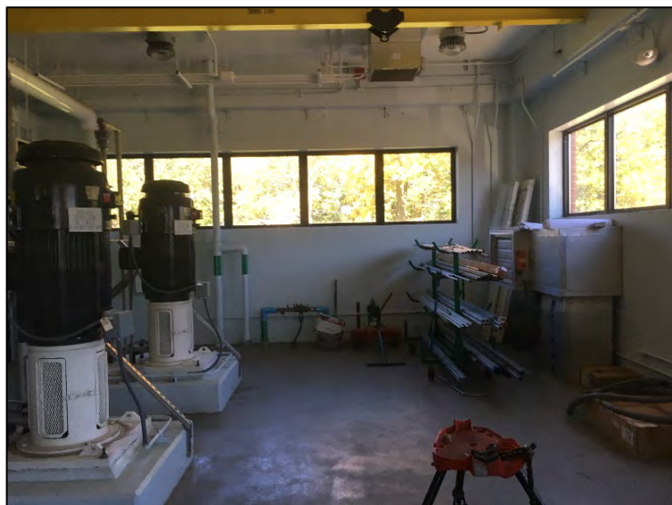
Figure 15. North Wall of East High-Service Pump Station
