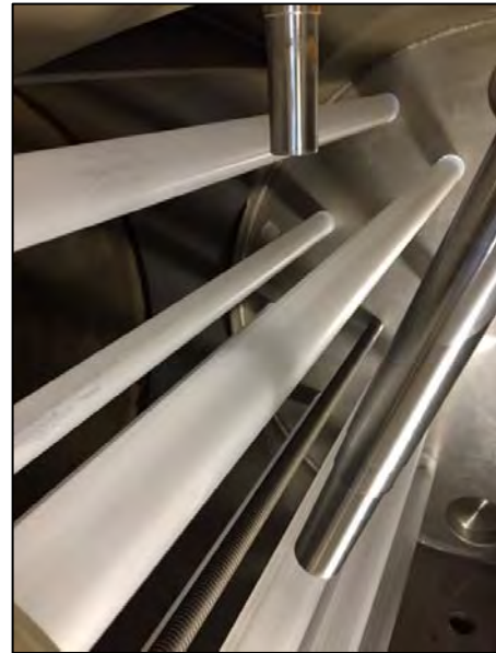
Figure 6. Example photograph of UV reactor quartz sleeves with calcium carbonate fouling
