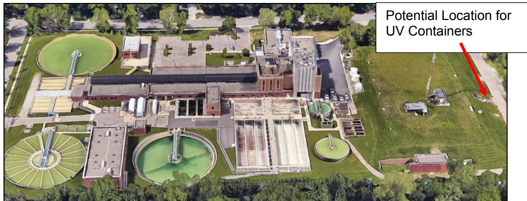
Figure 8. UV Containers Near Finished Water Reservoir
