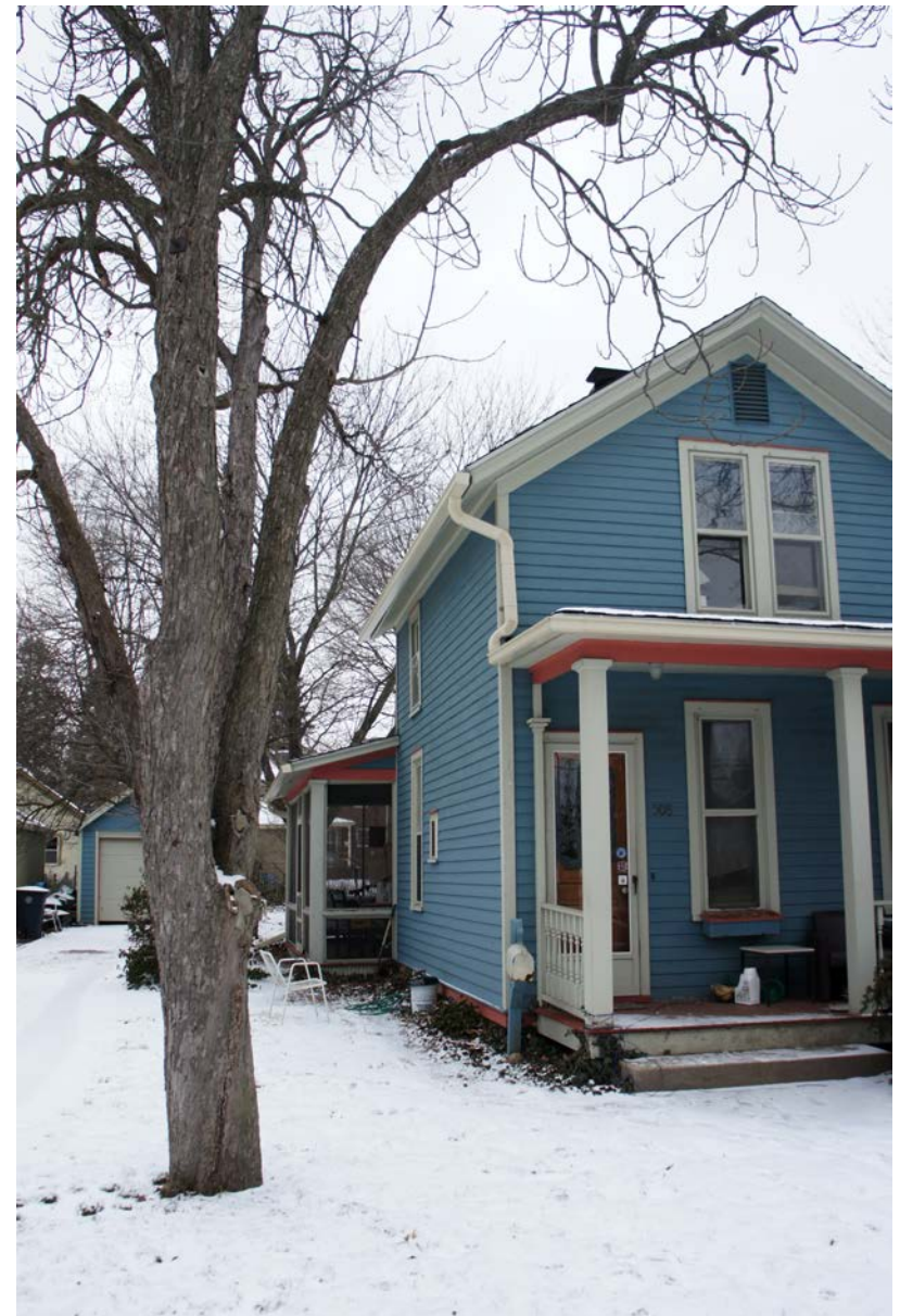
photo of front elevation (1980's era screened-in porch to be glassed in)
