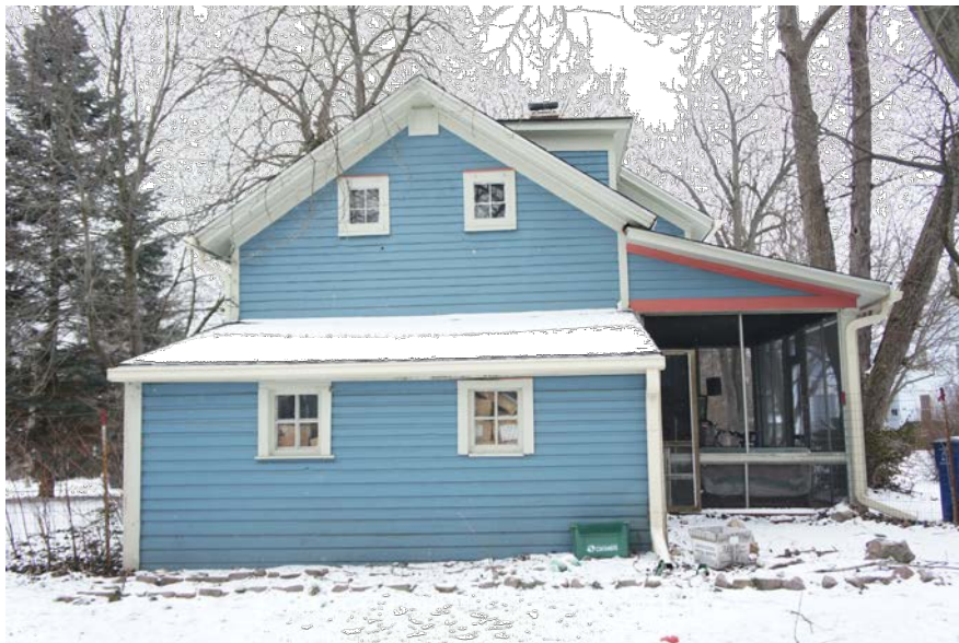
photo of west elevation (shed to be removed and replaced)
