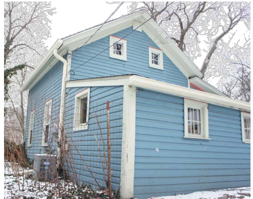
photo of north west elevation (shed to be removed and replaced)
