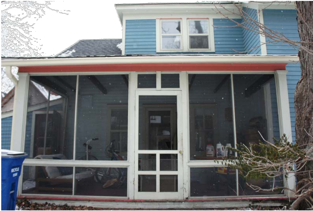
photo from south. (1980's era screened-in porch to be glassed in)
