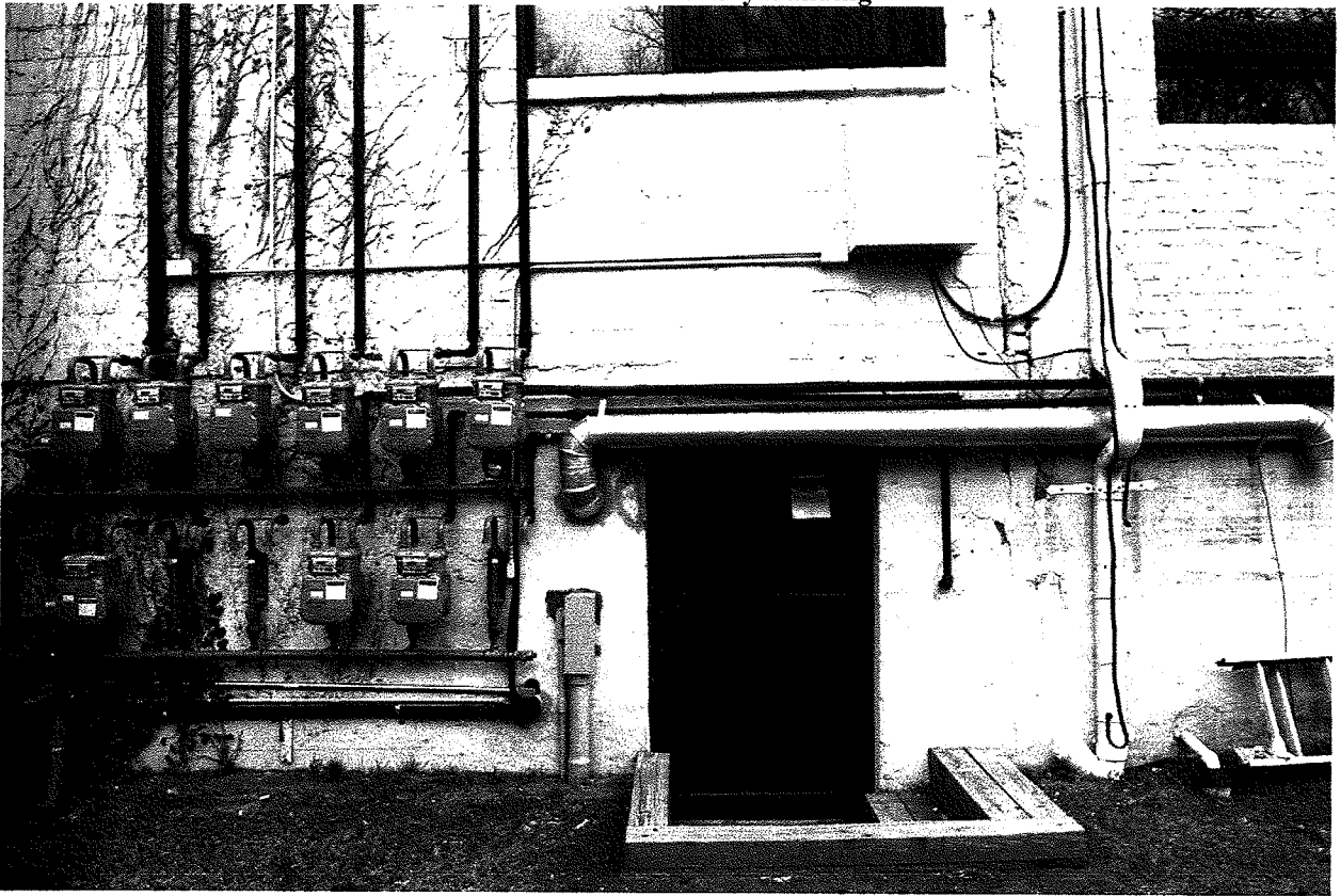
The Northern Brewery Building
