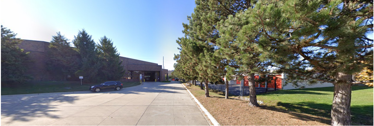
The AAATA property on South Industrial, left of the neighboring storage business. [ street view ]
