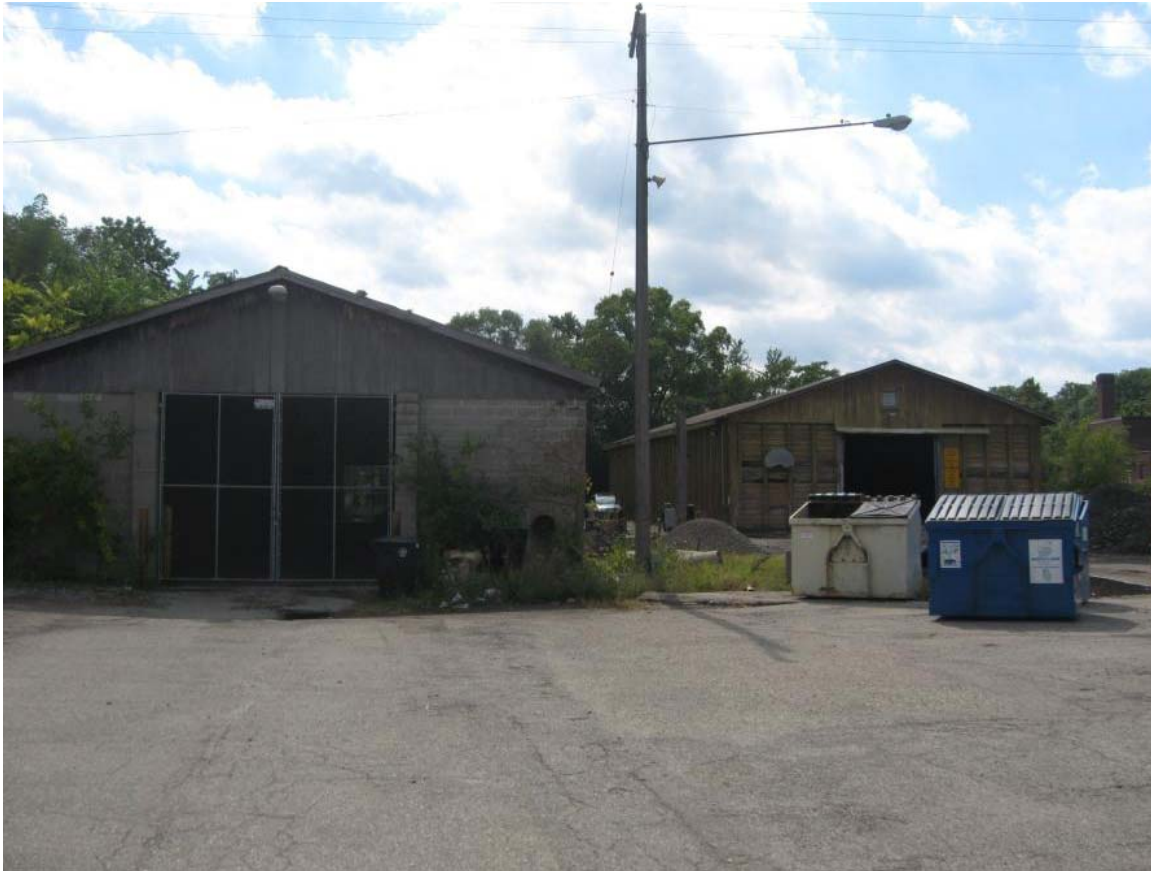
Garage & Salt Storage Buildings Within Floodway (Removal with FEMA Grant Pending)
