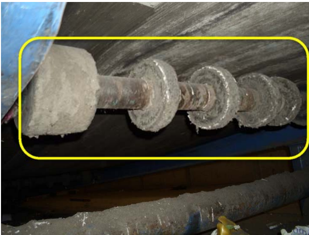
Return rollers need to be cleaned.
