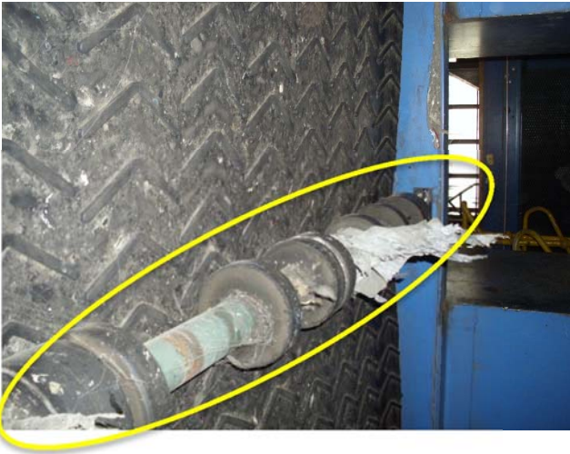
Return rollers are worn and wrapped, replacement required.
