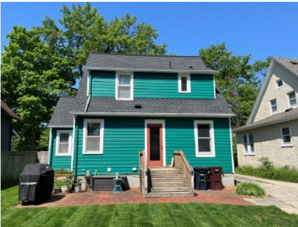
115 Crest Ave, rear, 2024 (courtesy of applicant)
