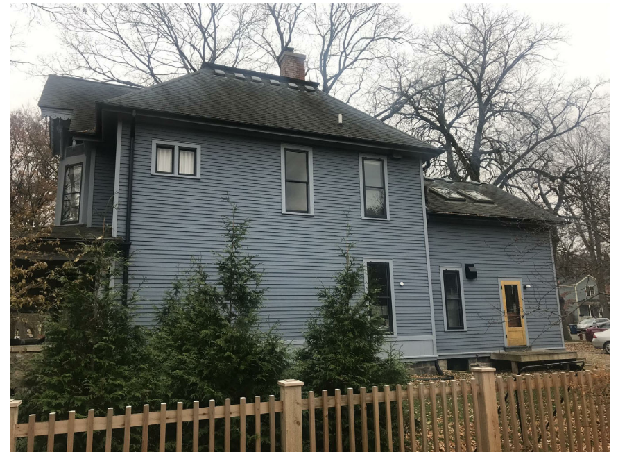
View of North Elevation
