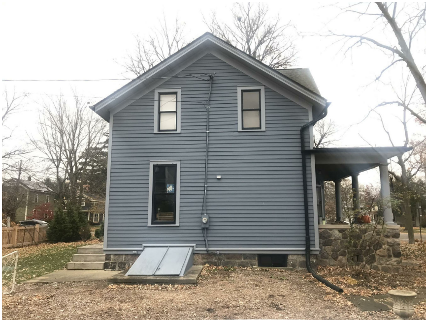
View of East Elevation
