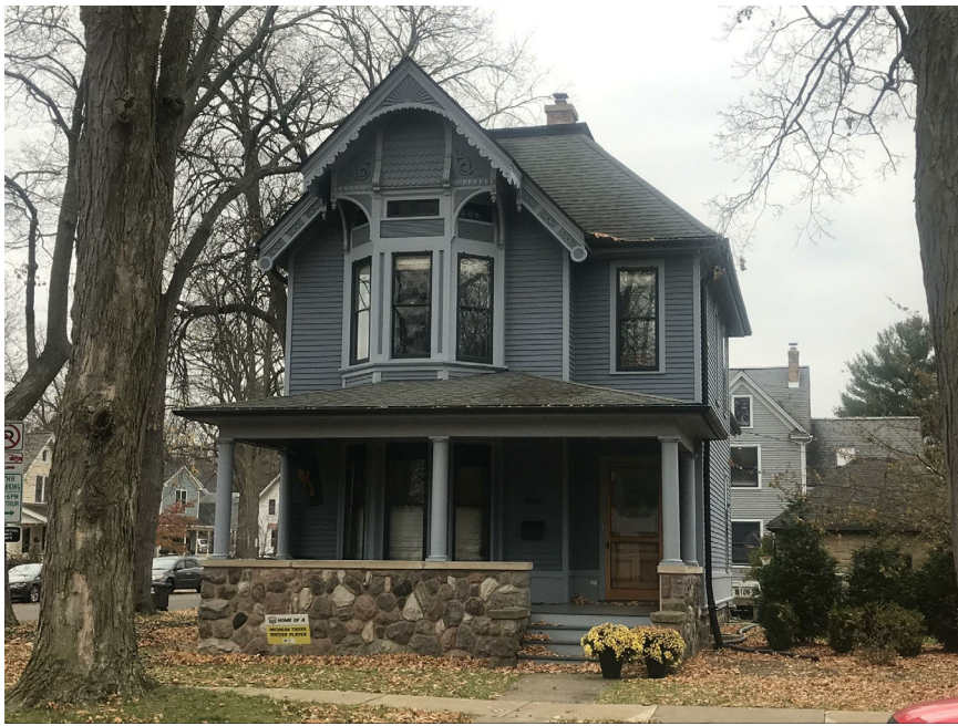
View of West Elevation
