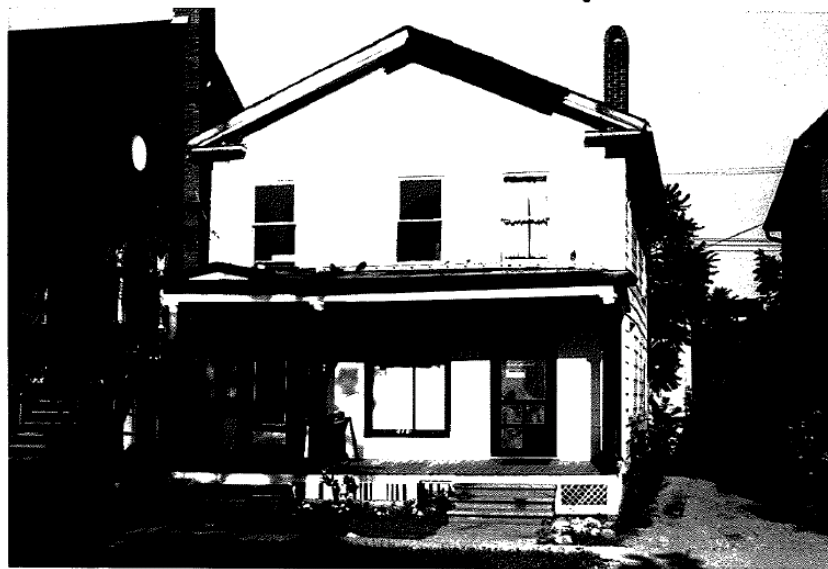
RESIDENCE OF EDWARD MUNDY, MICHIGAN'S FIRST LIEUTENANT GOVERNOR DURING THE ADMINISTRATION OF GOV. STEVENS THOMPSON MASON (1835-40) CONDEMNED - HOUSE DEMOLISHED SEPT. 22, 1975.
