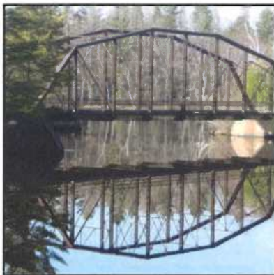
Upper Twin Falls Bridge, Dickinson County
