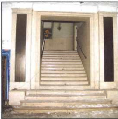
Fort Shelby Hotel, Detroit, Grand Stair, Before
