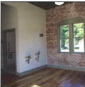
Boyne City Water Works Interior, After
