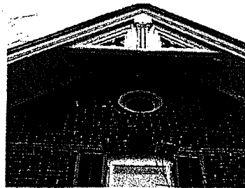
Fig. 12. West gable with stringcourse detail.
