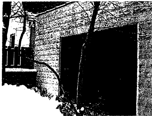
Fig. 4. Easternmost bay, original garage.
