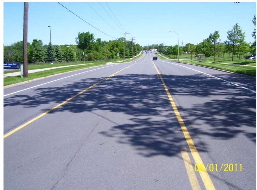
Green Rd 2011 Condition "Very Good"
