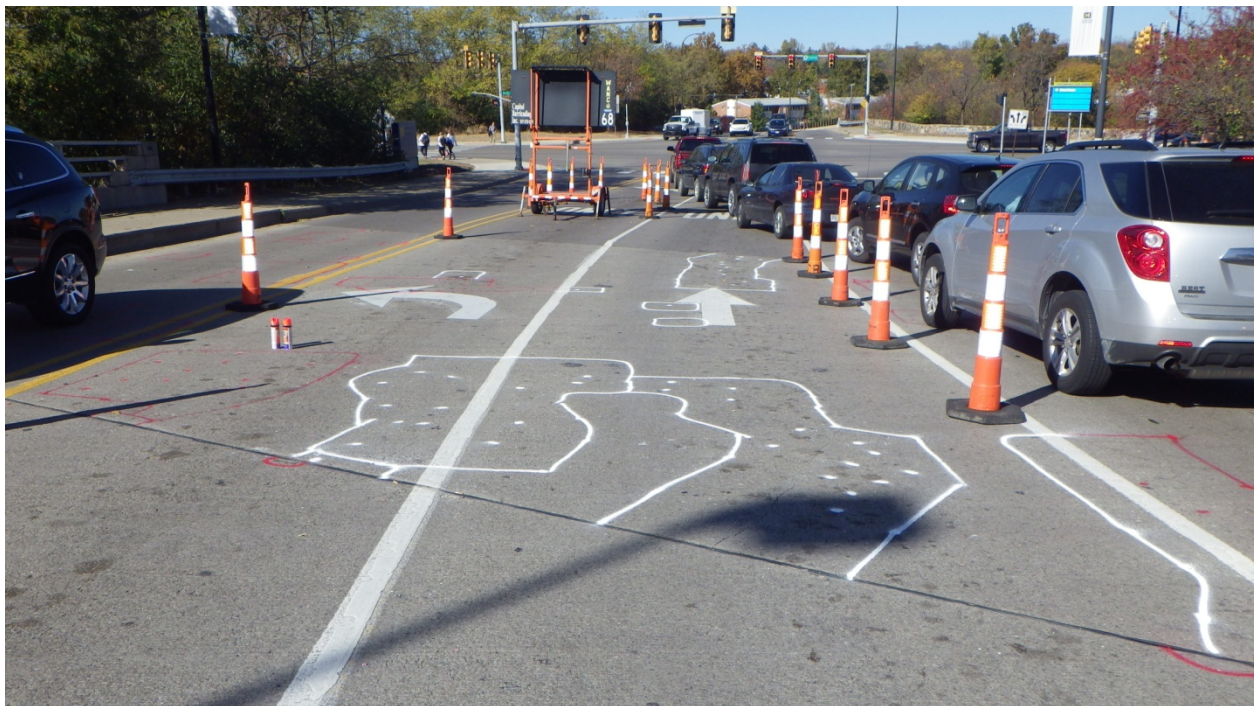
Figure 1 Deck Delaminations in North Span (looking north)
